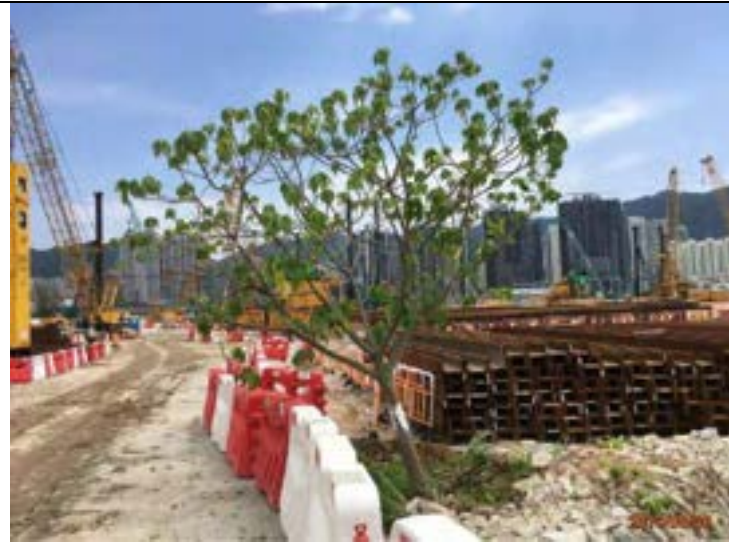
A32 Uprooted (after typhoon WIPHA – 31 July 2019)
