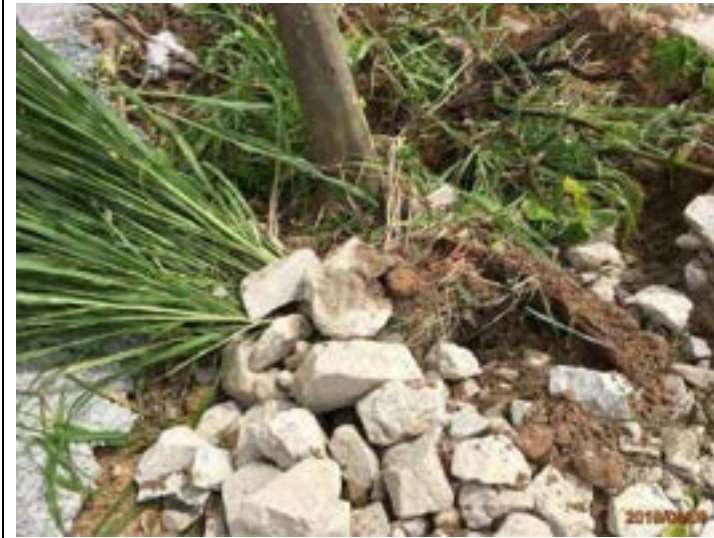
A32 Uprooted (after typhoon WIPHA – 31 July 2019)
