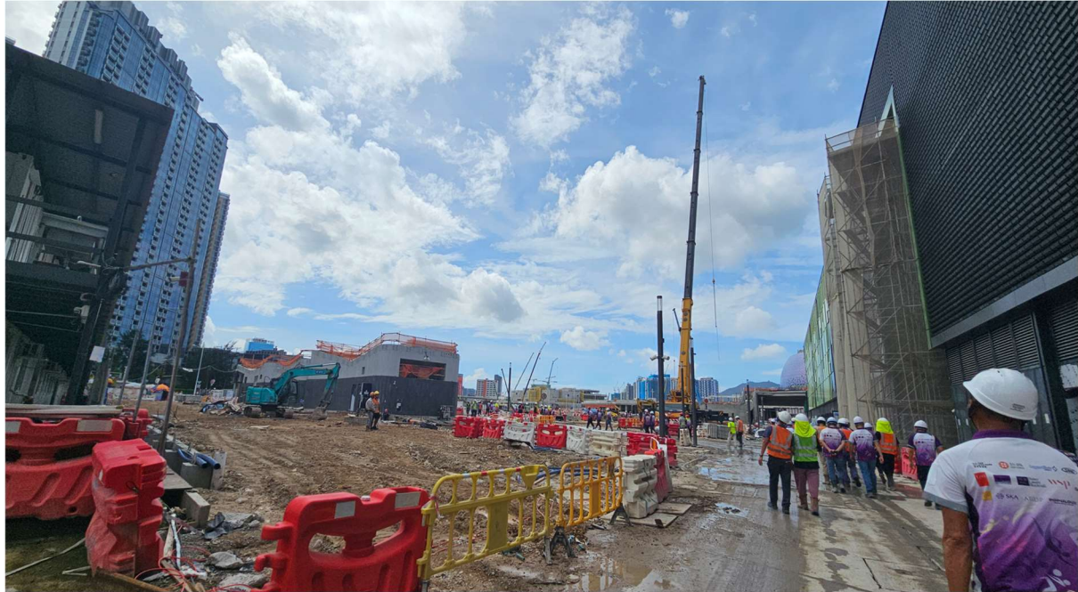
Photo 1: Regular site inspection carried out for checking dust mitigation measure on site. (25 June 2024)
