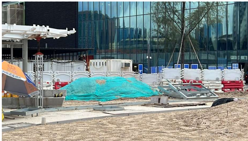
Photo 2: Covering sheet has been provided for stockpile on site.
