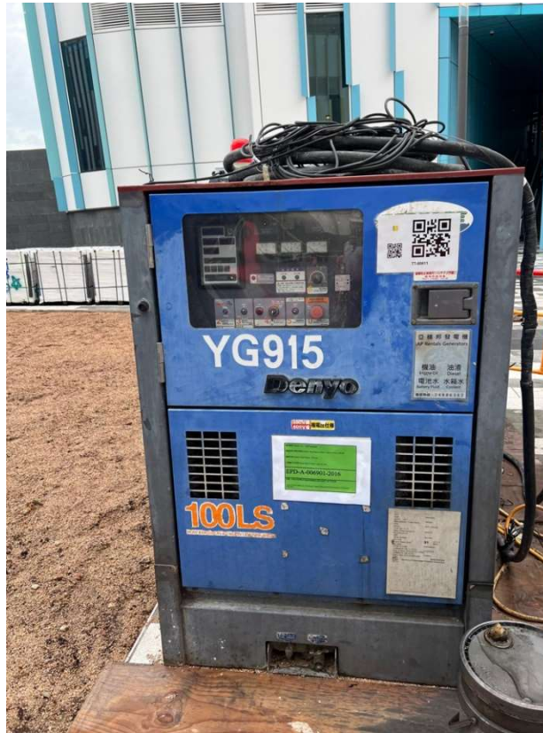
Photo 2: Power Mechanical Equipment with Quality Power Mechanical Equipment (QPME) labels were used at site to lower the noise nuisance to the nearby residents.
